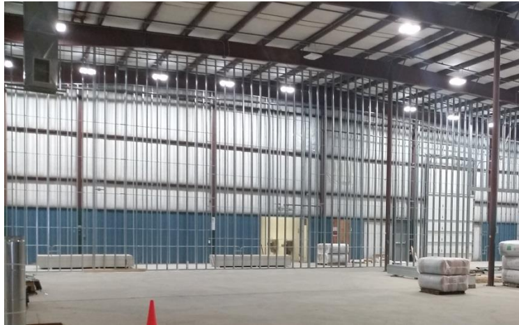
Preparing to create Clean Rooms
