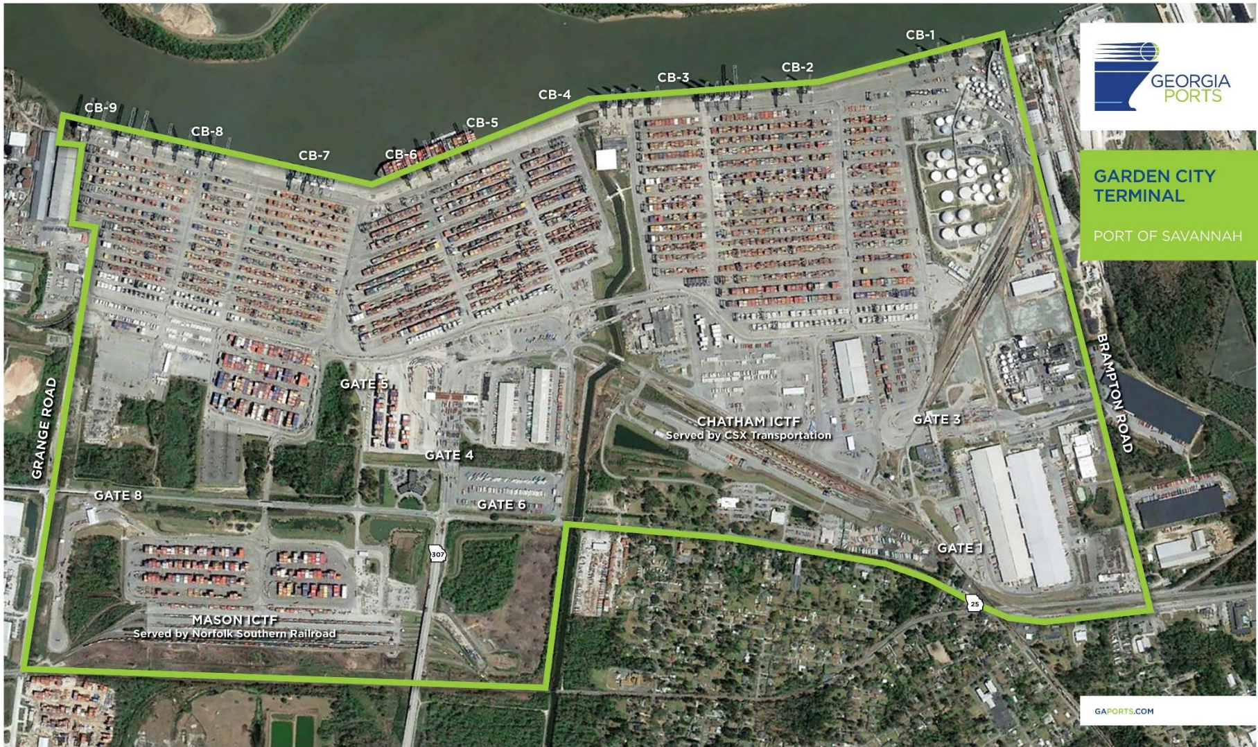
Garden City Terminal is owned and operated by the Georgia Ports Authority • V.Jun-2018
